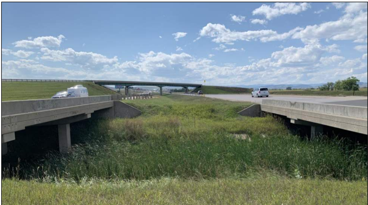
View west toward the Highway 1416 Bridge over I-90, from I-90.
